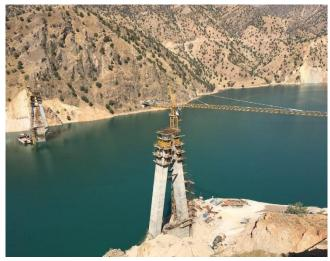
Sebalootak Bridge provides the access road for residents who parted away after the Third Dam over the Karoon River was dammed the river and submerged the existing road. The bridge spans over the dam reservoir. With a main span of 260m, it holds the title of the longest span cablestayed bridge in Iran till date. The total height of the longer pylon is around 100m from the ground. The water level in the dam lake varies from 800m to 845m.
