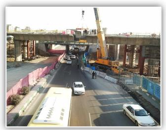
Jenah Intersection Bridges aim to facilitate transportation of vehicles in the intersection of two major highways in western Tehran. There are six bridges including two main bridges and 4 directional ones. The current of the available terrific did not obstruct during construction. Construction of nearly 25,000 m² of deck lasted a little more than two years.
