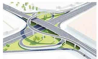
Najafi Intersection Bridges are located in the city of Hamedan in Iran. This combination of bridges consists of one main bridge that is stretched in North-South Direction and one directional bridge that facilitate the transportation of vehicles from the west to the north, passing over the main bridge.
