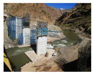
Doab River Bridge is constructed over a dam reservoir in order to recover a submerged bridge that used to provide residents of a couple of villages and small towns with a local access road. The bridge was constructed before watering of the dam, which created the possibility of construction of piers at a distance of 30m and avoiding very long spans over the entire lake width.
