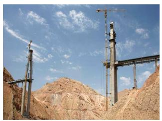
Lali Cable-Stayed Bridge provides the access road for residents who parted away after the Gotvand Dam over the Karoon River was constructed. The bridge spans over the dam reservoir. The total height of the pylons is around 146m from the ground.
