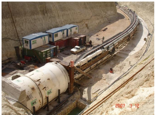
Assembly of Herrenknecht Model S-124 in its previous job
