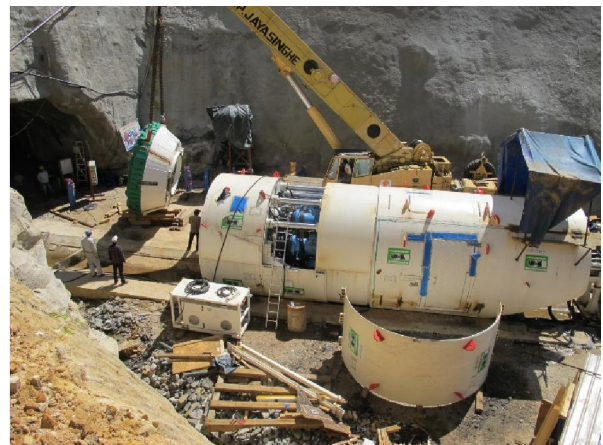
Assembly of first TBM at exit of Dyraaba headrace Tunnel
